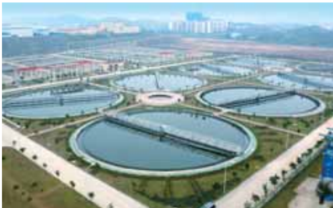
Chongqing Tangjiatuo Waste Water Plant
