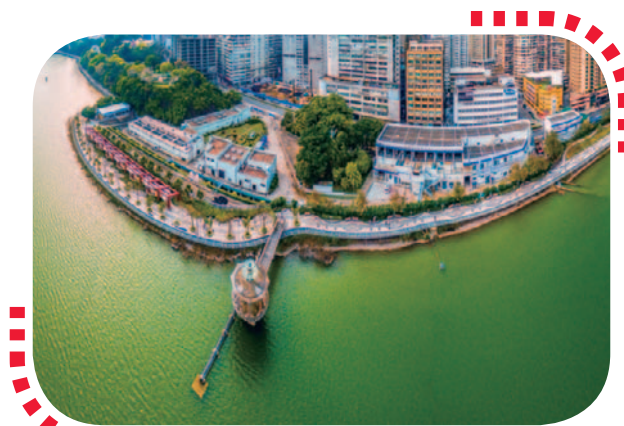
Macau Water Plant
