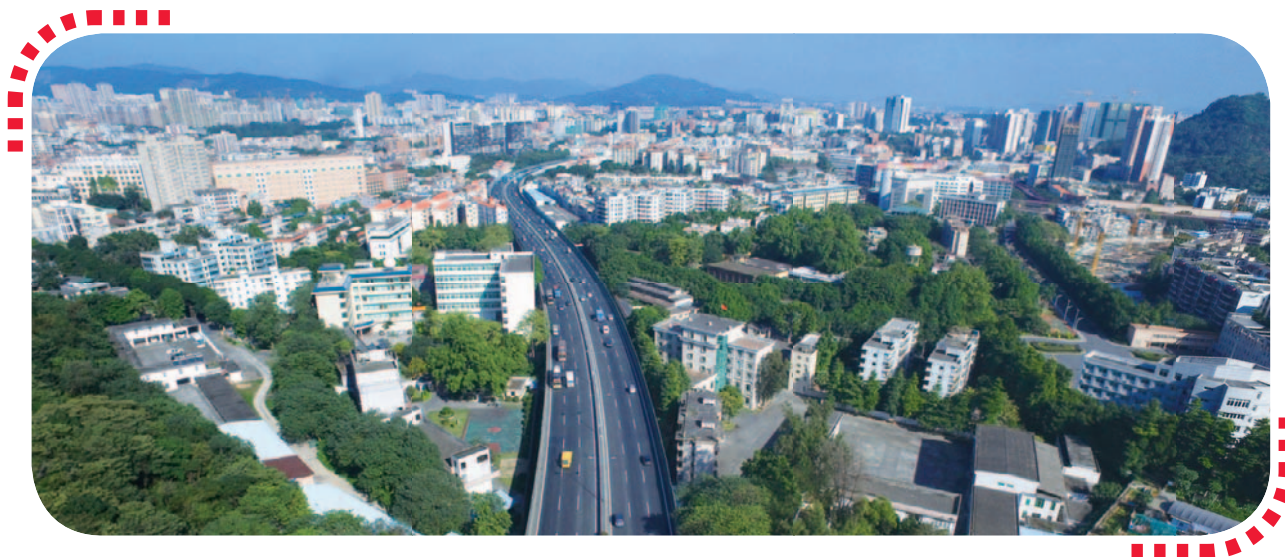
Guangzhou City Northern Ring Road
