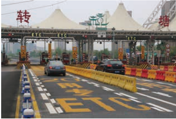
ETC system applied on Hangzhou Ring Road
