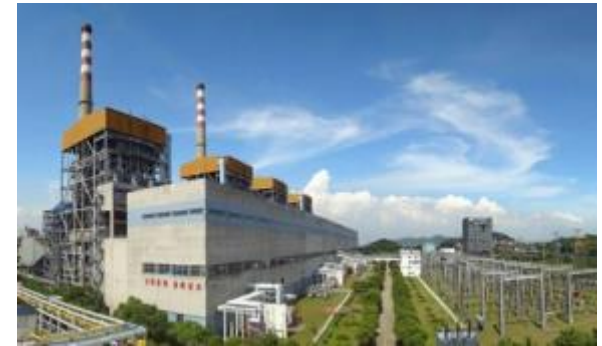
Zhujiang Power Plant
