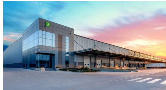
Single Level Warehouse
