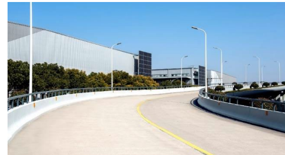
Ramp Access to Double Level
