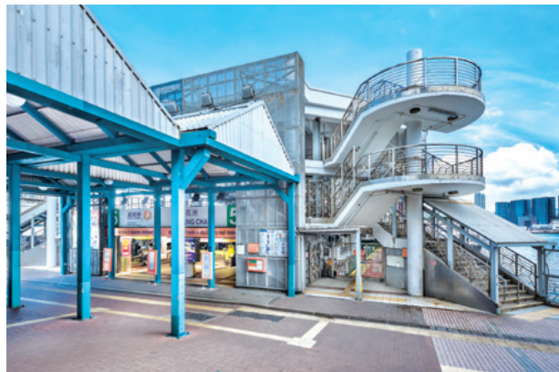
AEDs are installed at selected NWFF ferry piers to strengthen safety of our passengers.
