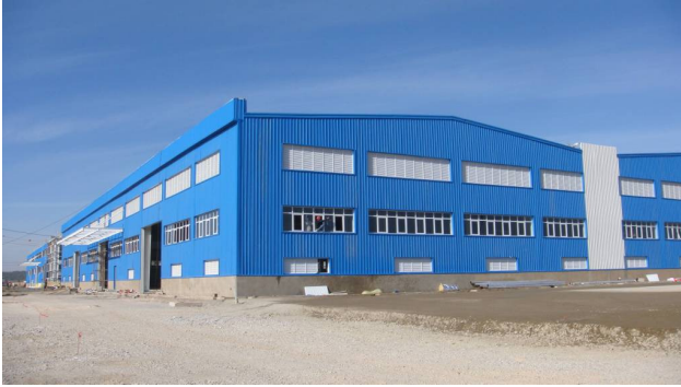
Photo 3: Warehousing facilities in Kunming Terminal commenced operation in early 2010.
